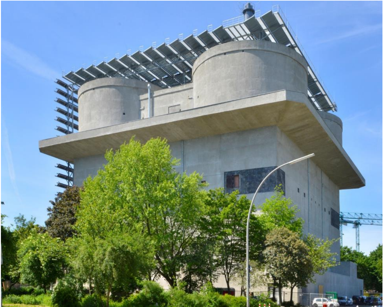
Abb. 6 Der Energiebunker in Hamburg Wilhelmsburg (Foto © Ariane Ruff)
