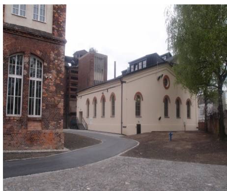
Obr. 53 Kompressorovna – Compress Hall
